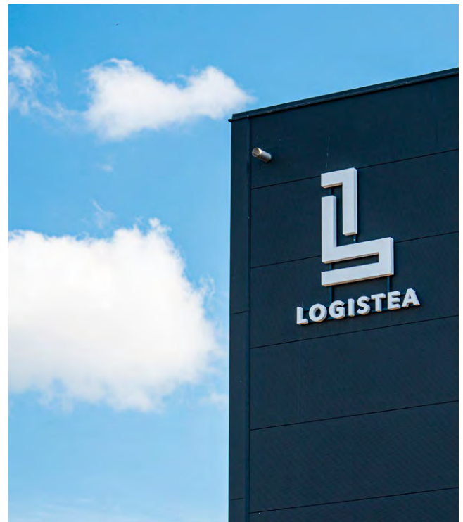
Logistea's property Vindan 1 in Borås is certified according to BREEAM In-Use Very Good level.
